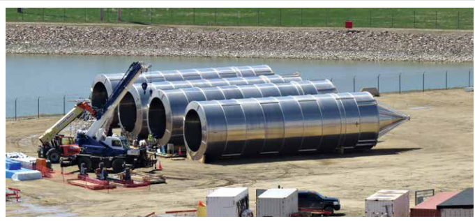
After manufacture in Germany, light-weight aluminum polyethylene pellet loading blenders were shipped to the site for assembly and specialized welding.
