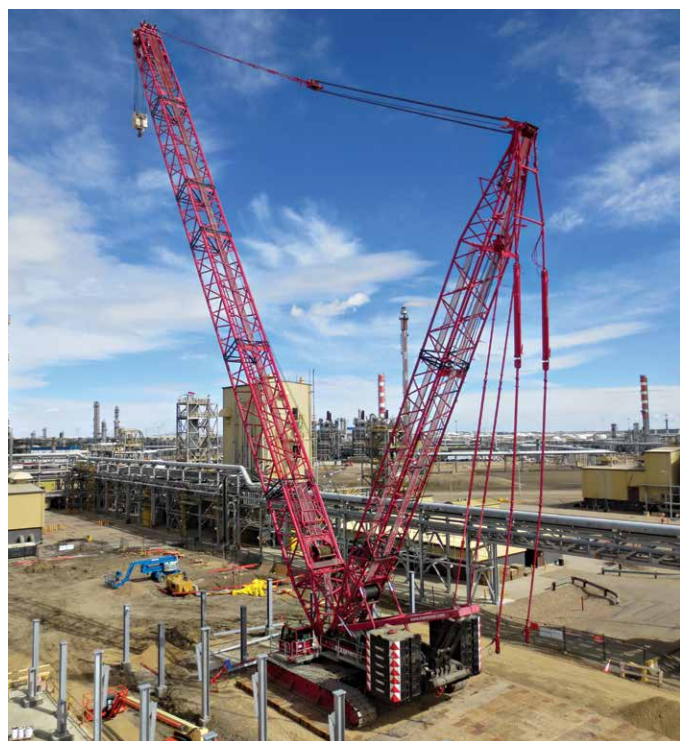
The installation of piperacks and other structural modules manufactured off site continues.
