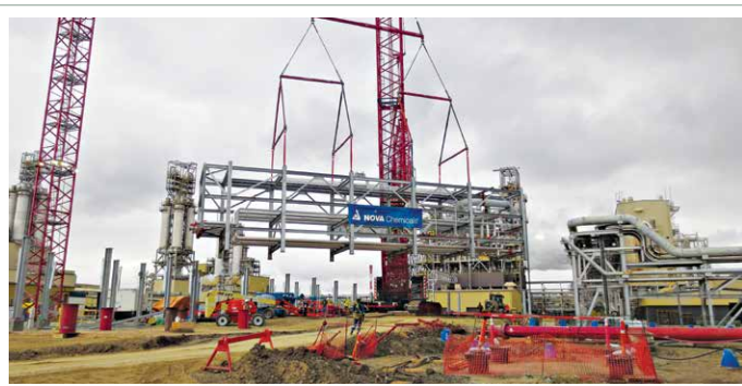
On April 16, 2014 the first piperack module was safely delivered and set into place. This was the first of 51 modules to be shipped from Ledcor's modular assembly yard in Nisku. The last module is scheduled for shipment in early 2015.
