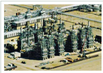
Aerial view of E2. Furnace refurbishment is underway regardless of whether we proceed with E2DB.
