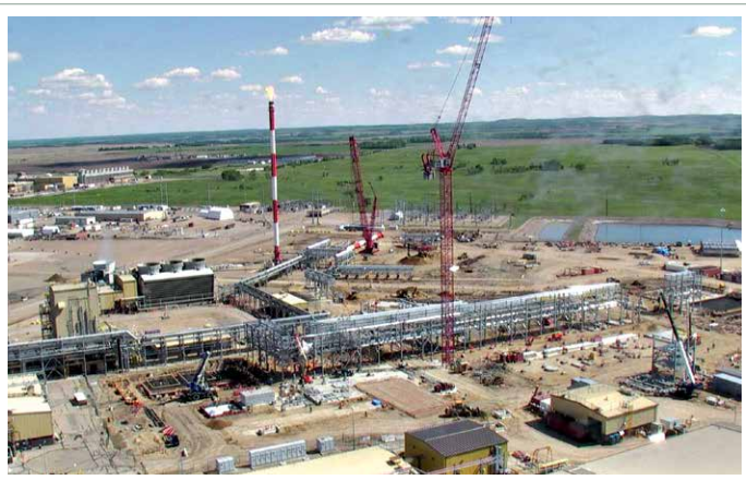
A view of the expansion area as of June 2014.
